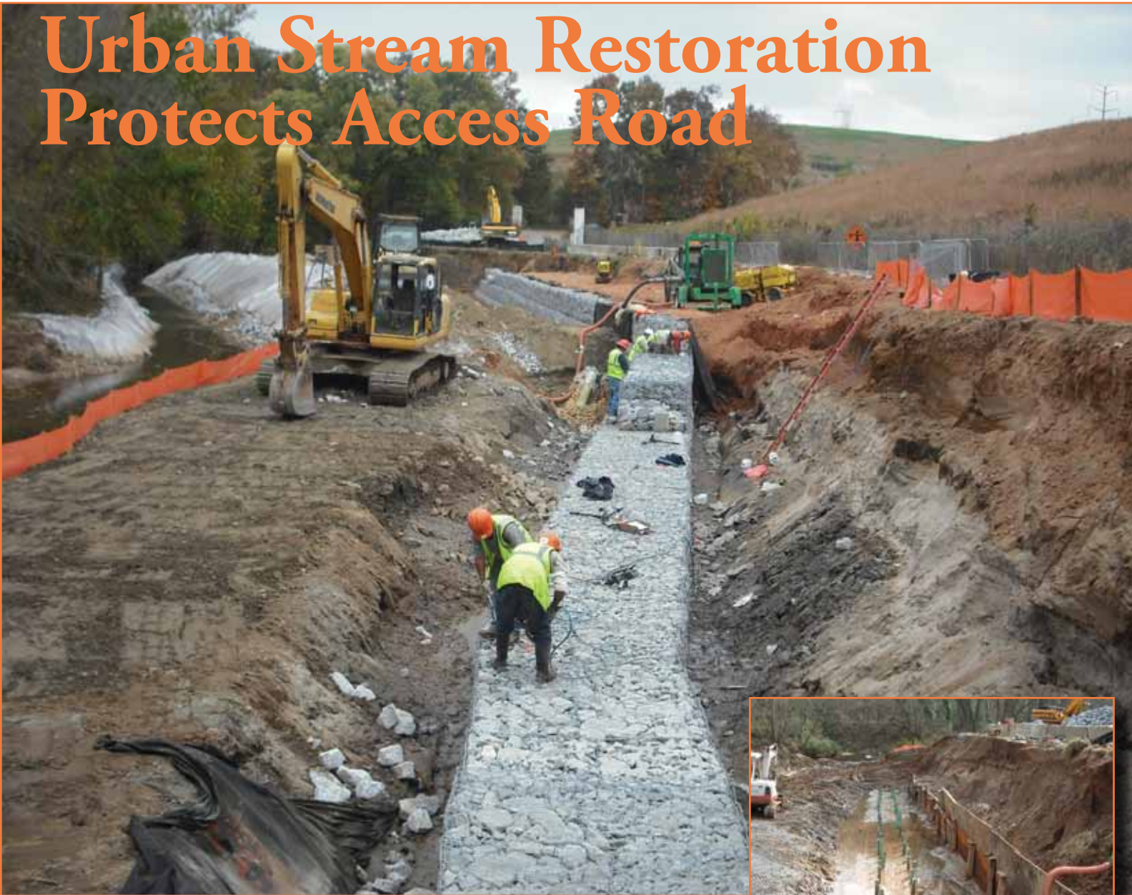
Workers install gabion baskets (above). Concrete foundation poured and ready for gabion basket installation (inset).
