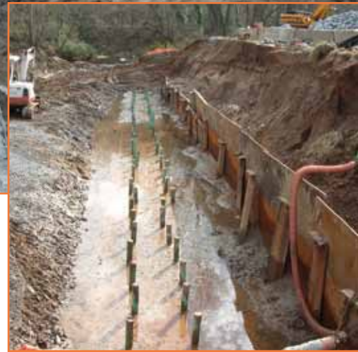
Workers install gabion baskets (above). Concrete foundation poured and ready for gabion basket installation (inset).
